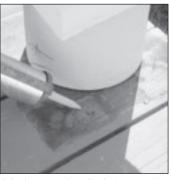
**4.** Apply construction adhesive\* to top and bottom surfaces of column.
