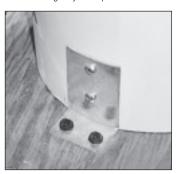
**6.** Mark and drill holes in floor and column shaft for corner/ angle brackets (not included). (HB&G column installation kit available #17040)
